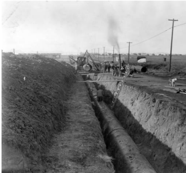
Sewer crew laying clay line in trench. 1923
