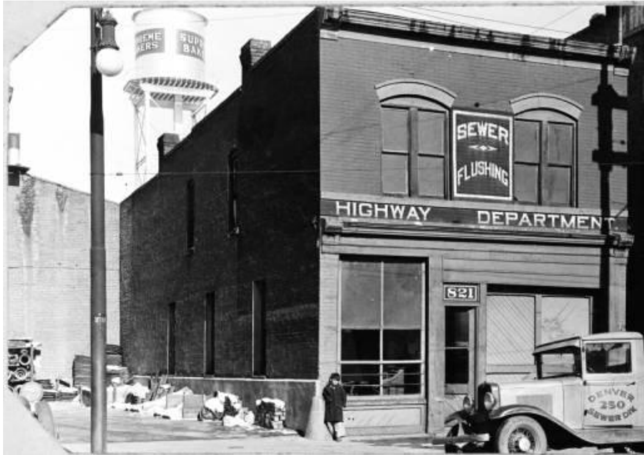
Sewer Flushing Department of the Denver Highway Department. Circa 1930 - 1940 Photo Courtesy of Denver Public Library, Western History Collection, Reference X - 20715
