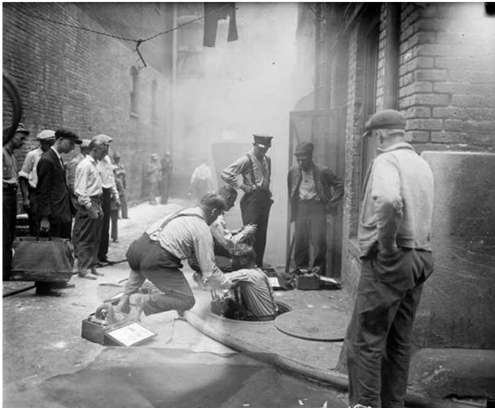
Sewer crew coming out of a manhole in Denver. Circa 1920 - 1940 Photo Courtesy of Denver Public Library, Western History Collection, Reference Rh-1462
