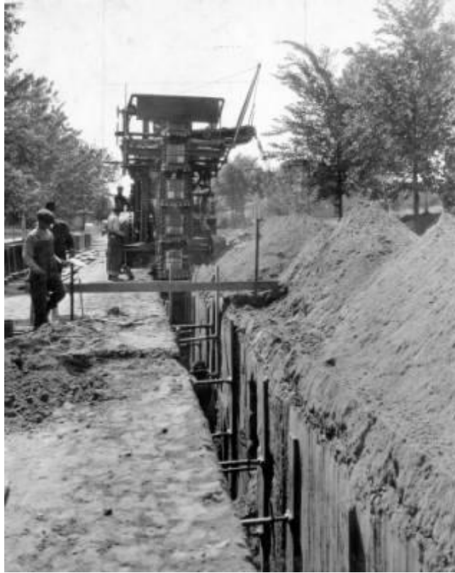
Trench digging machine. Circa 1910 - 1920
