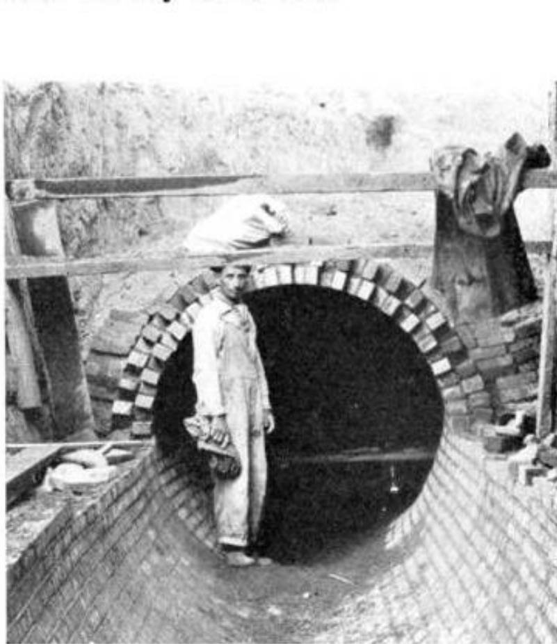
Sixty-inch circular sewer, two rows of bricks North Denver Storm Sewer
