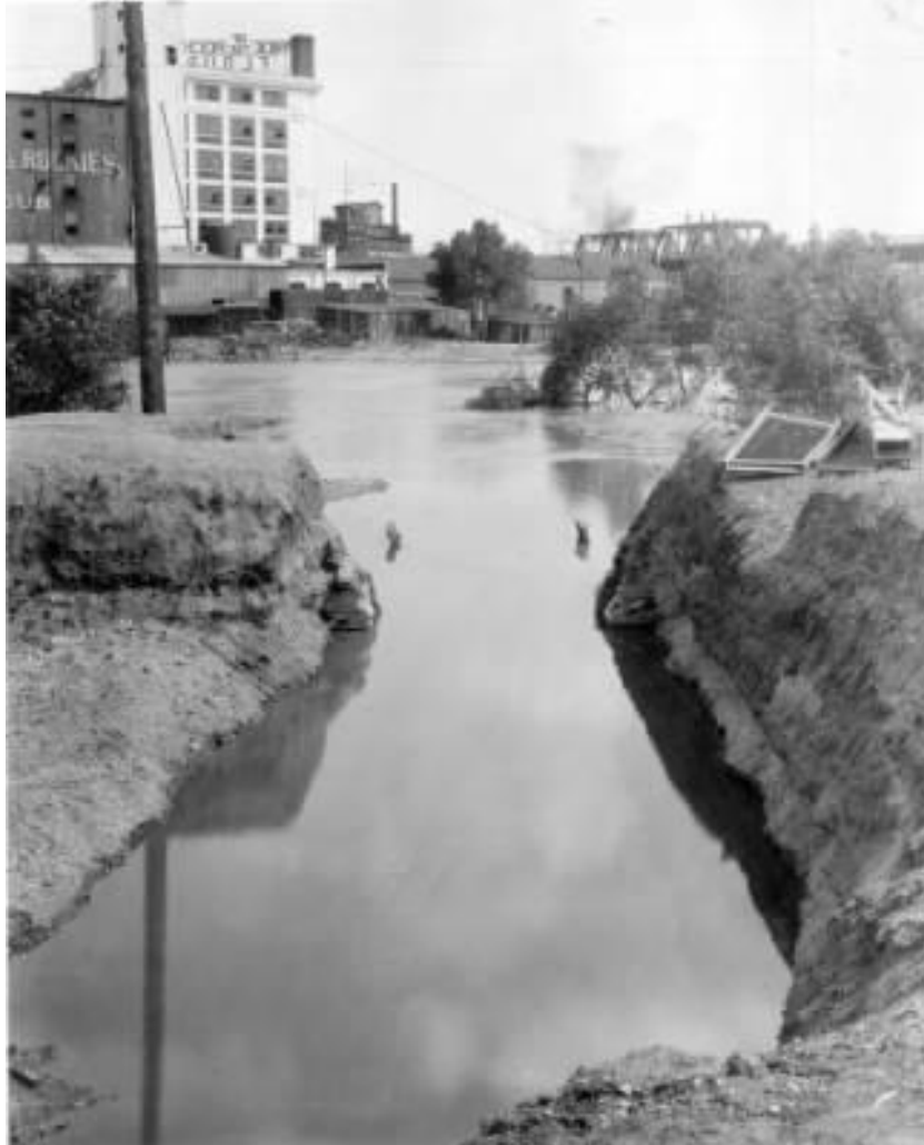
View of a ditch leading to the South Platte River during construction of the twin conduits for the North Denver Storm Sewer #2, Circa 1910-1920.
