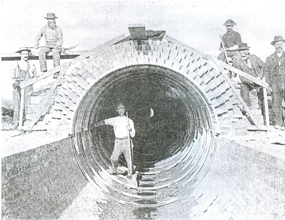
Delgany Street Sewer Extension. 1895
