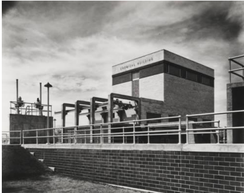
Chemical Building at the Metropolitan Denver Sewage Disposal District Sewage Disposal Plant, 1937. Photo Courtesy of Denver Public Library, Western History Collection, Reference Z-10068
